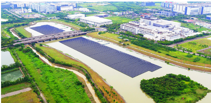
AUO Installed a 6 MW Floating Power Plant at the public flood retention ponds No.1 and No.2 in Tainan
